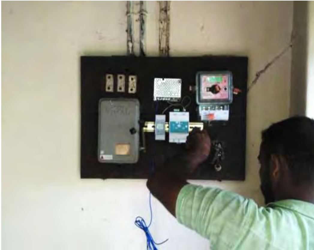
Figure 15: Data logger: Smart meter and data logger being fixed in a 1BHK home in Kalamassery, South Aluva. The unit measured the consumption every second and logged the parameters into a memory device. The unit along with the data was extracted after a month. The extracted data was subsequently analysed while the unit was attached in another home.
